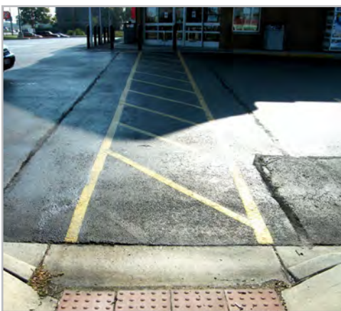
The sidewalk (top) allows pedestrians to avoid walking through access aisles. Striping is another method to highlight pedestrian travel through parking lots (bottom). Sources: NNECAPA, Lexington, MA (top); MORPC, Columbus, OH (bottom).
