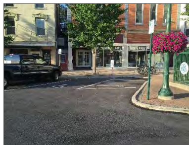
Northeast Public Square Lot – One (1) ADA compliant space with an accessible aisle and dedicated curb ramp.
