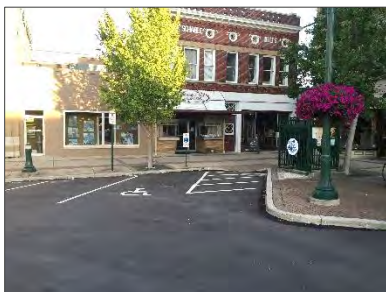
Southeast Public Square Lot – One (1) ADA compliant space with an accessible aisle and dedicated curb ramp.
