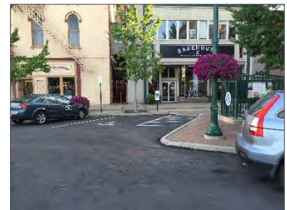
Southwest Public Square Lot – One (1) ADA compliant space with an accessible aisle and dedicated curb ramp.
