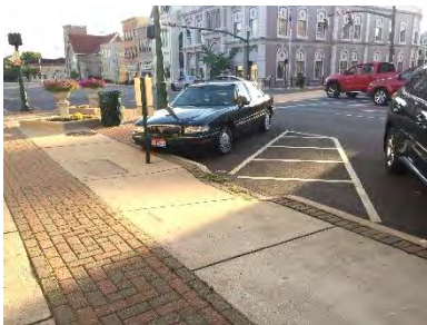
Market Street (Block 8) – The handicap space meets ADA requirements.
