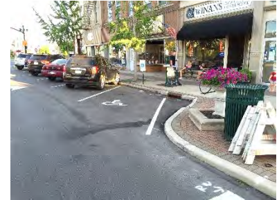
Main Street (Block 7) – The handicap space does not provide an ADA compliant accessible aisle.
