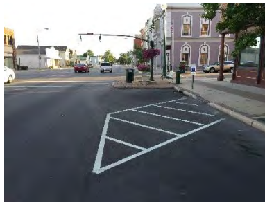
Market Street (Block 7) – The handicap space meets ADA requirements and could be considered a van accessible space.
