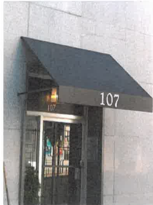
FABRIC-WRAPPED ALUMINUM AWNING: VENETIAN-STYLE ALUMINUM FRAME w/ BLACK SUNBRELLA FABRIC
