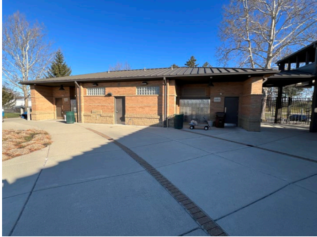
Men's/Women's View of locker Room
