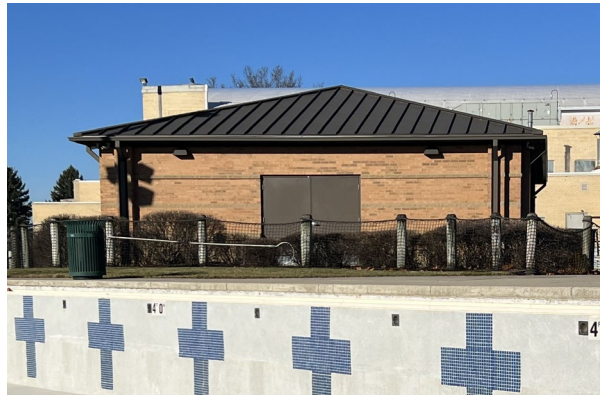
Pool Equipment Building
