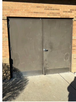
Exterior Doors at Pool Mechanical Building
